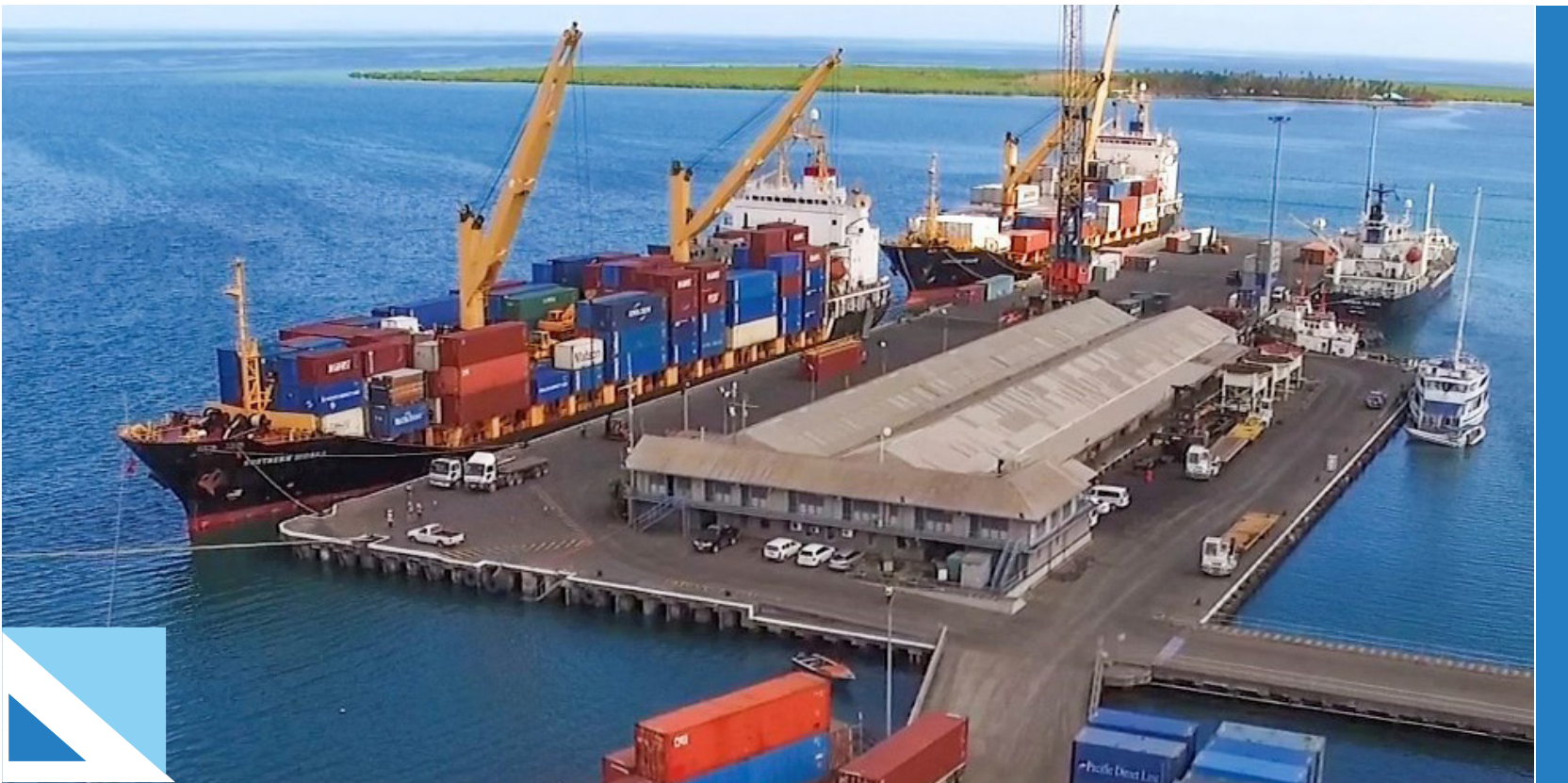
Aerial view of Port of Lautoka undergoing wharf rehabilitation works
