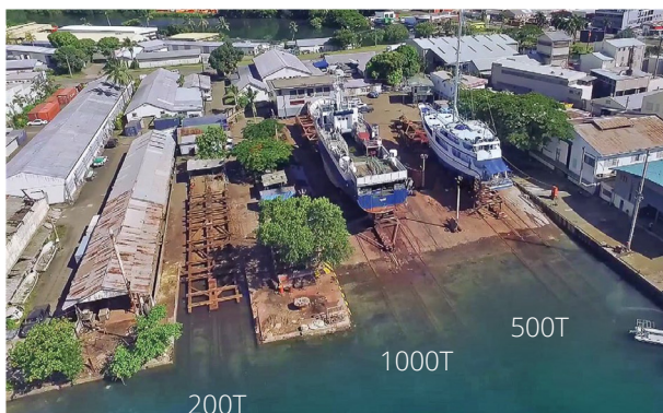
FSHIL 200T, 500T & 1000T Slipways
