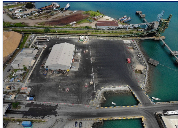
Lautoka Container Yard 3 - After Completion
