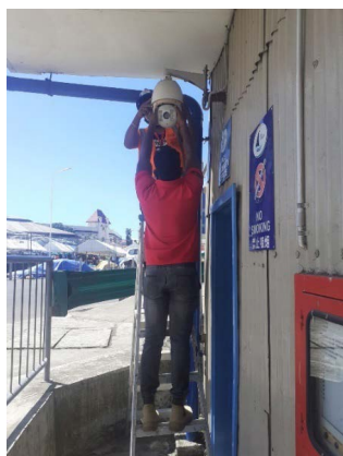
CCTV cameras being installed at the Port of Suva
